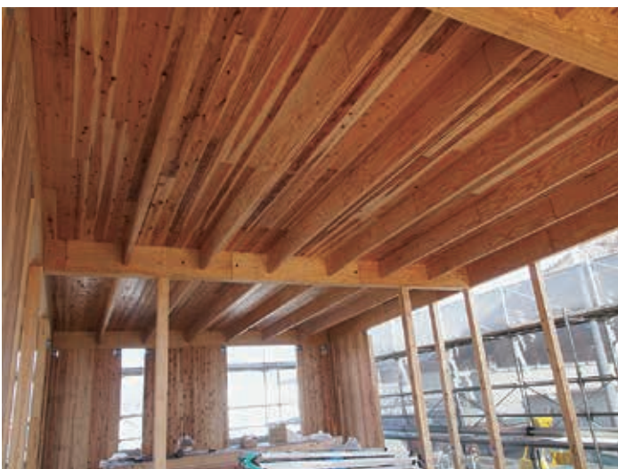
Ceiling used LVL and CLT
