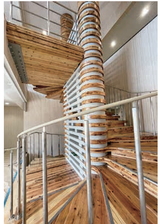
Stairs made of wood and concrete
